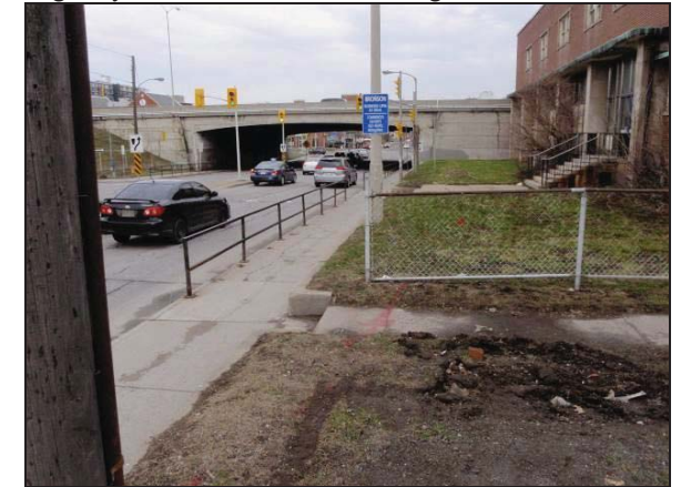
Plate 40: Southeast view of SE quadrant of Highway 417/Bronson Avenue bridge.
