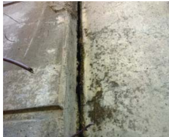
Photo 02: Cork asphalt board in expansion joint
