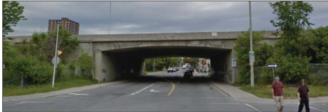
Figure 16. Booth Street Bridge (looking north)
