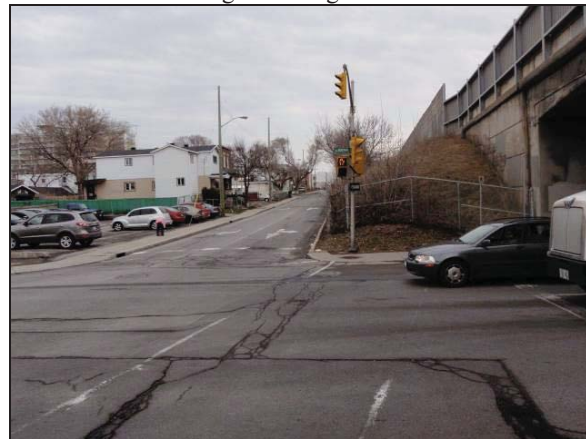
Plate 34: East view of NE quadrant of Highway 417/Booth Street bridge at Raymond Street.
