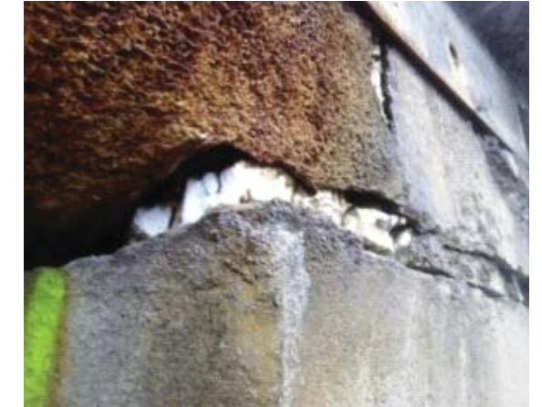
Photo 02: Polystyrene Expansion Joint
