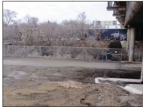
Plate 21: West view of building at SW quadrant of Highway 417/ O-Train bridge from SE quadrant.
