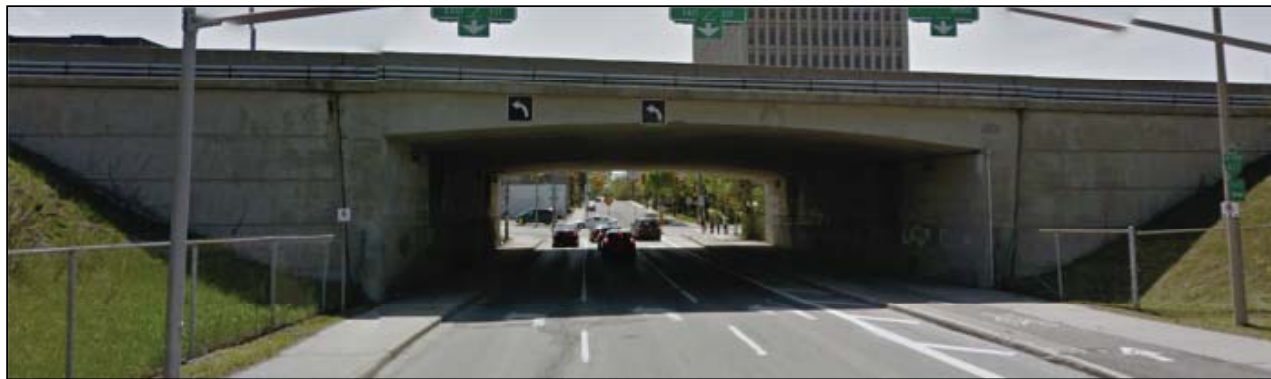
Figure 25. O'Connor Street Bridge (looking south)
