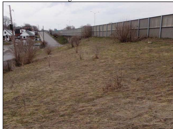
Plate 12: West view of SE quadrant of Highway 417/ Fairmont Avenue bridge.
