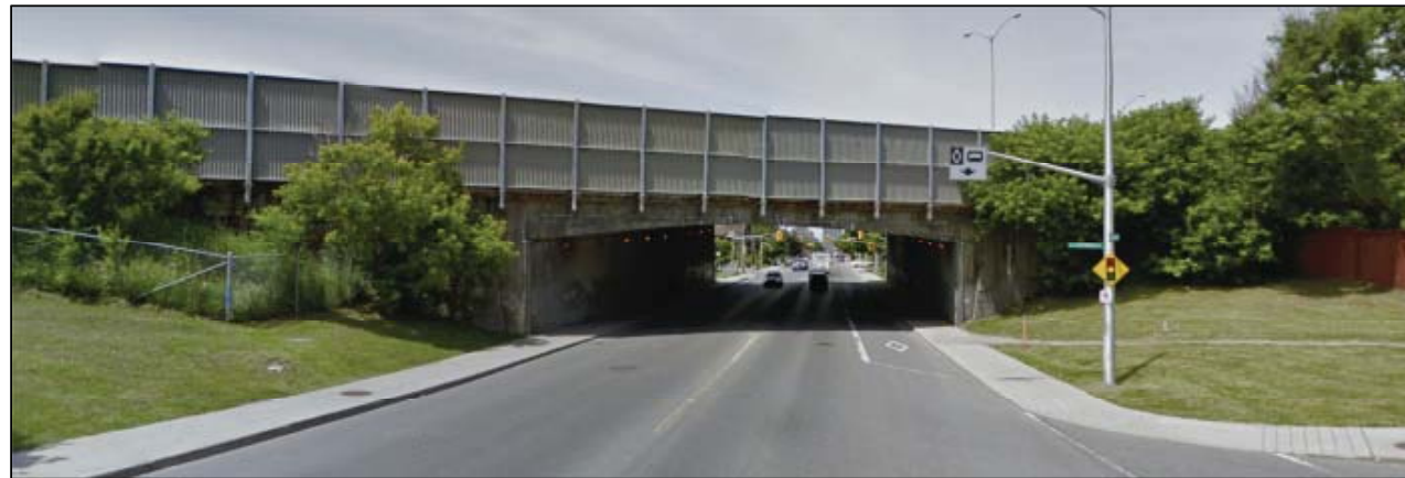
Figure 1. Holland Avenue Bridge (looking north)
