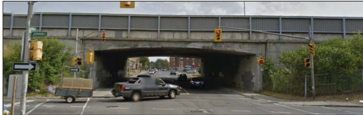
Figure 17. Booth Street Bridge (looking south)
