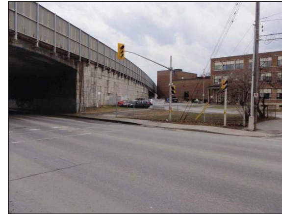
Plate 1: West view along north side of highway west of Holland Avenue.
