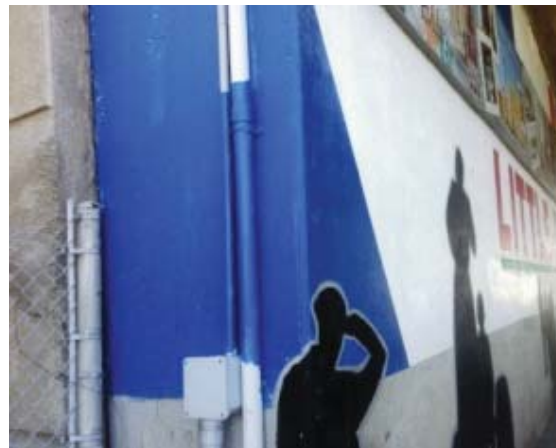
Photo 01: Paint on abutment walls
