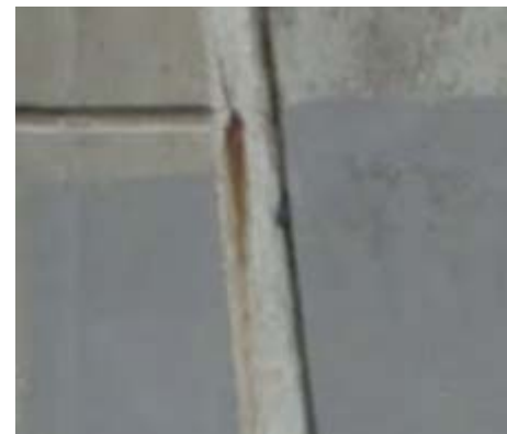
Photo 02: Cork asphalt board in expansion joint
