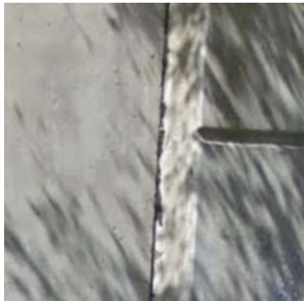
Photo 01: Cork asphalt board in expansion joint
