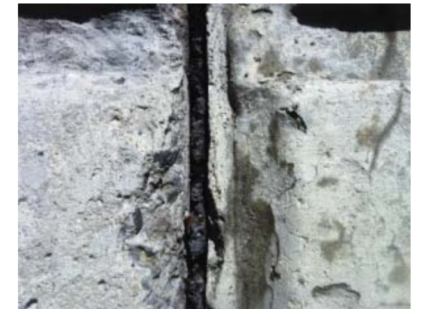
Photo 02: Cork asphalt board in expansion joint
