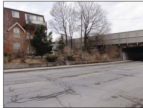
Plate 15: West view of SW quadrant of Highway 417/ Bayswater Avenue bridge.
