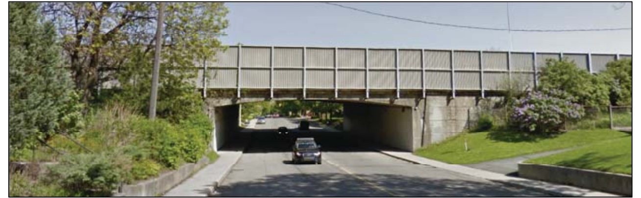
Figure 7. Bayswater Avenue Bridge (looking north)
