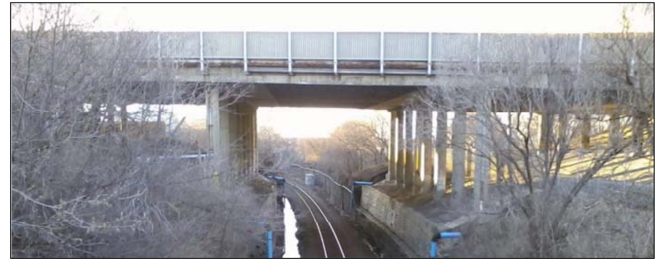
Figure 11. O-Train Bridge (looking north from pedestrian bridge)
