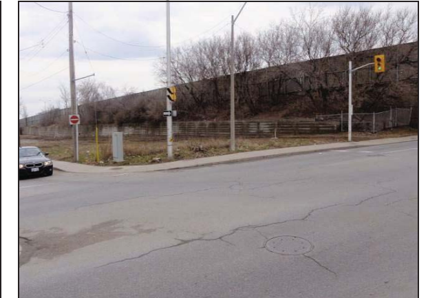
Plate 6: Southeast view of NE corner of Highway 417/ Parkdale Avenue bridge.
