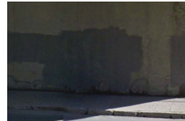
Photo 01: Paint on abutment walls
