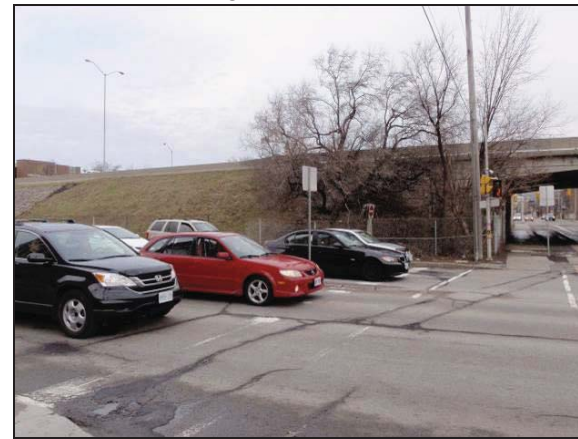
Plate 51: Northwest view of SW quadrant of Highway 417/ O'Connor Street bridge.
