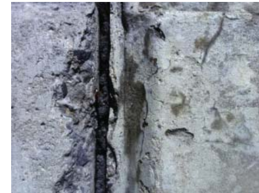
Photo 01: Cork asphalt board in expansion joint
