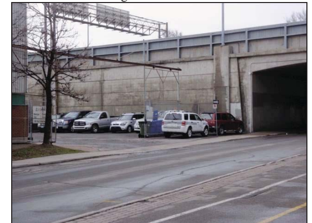
Plate 42: Southeast view of NE quadrant of Highway 417/Percy Street.
