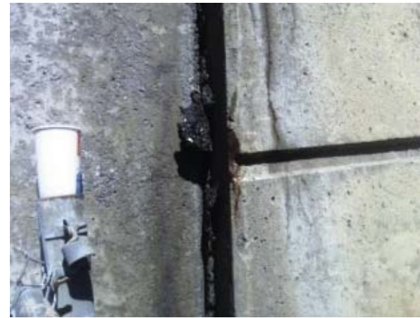
Photo 02: Cork asphalt board in expansion joint
