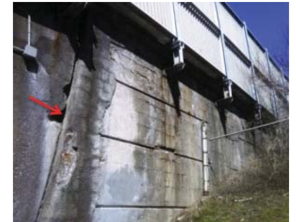
Photo 02: Cork asphalt board in expansion joint
