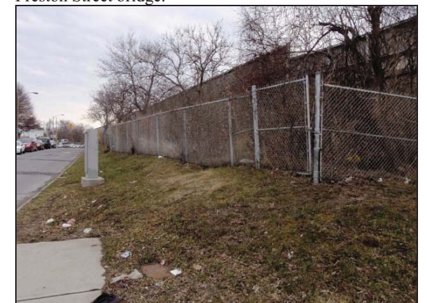
Plate 30: East view of NE quadrant of Highway 417/ Rochester Street bridge at Raymond Street.
