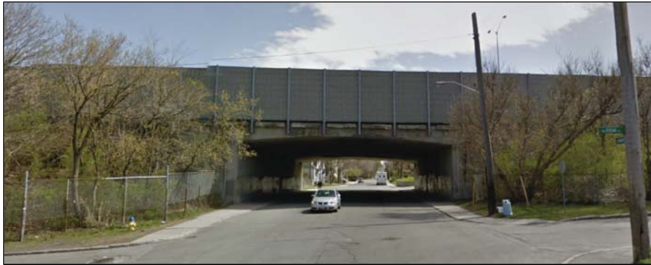
Figure 6. Fairmont Avenue Bridge (looking south)
