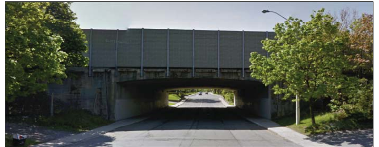
Figure 8. Bayswater Avenue Bridge (looking south)
