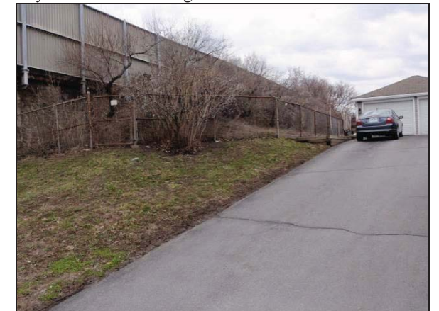
Plate 16: East view of SE quadrant of Highway 417/ Bayswater Avenue bridge.
