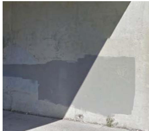
Photo 01: Paint on abutment walls
