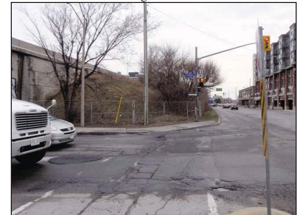
Plate 52: East view of SE quadrant of Highway 417/ O'Connor Street bridge.
