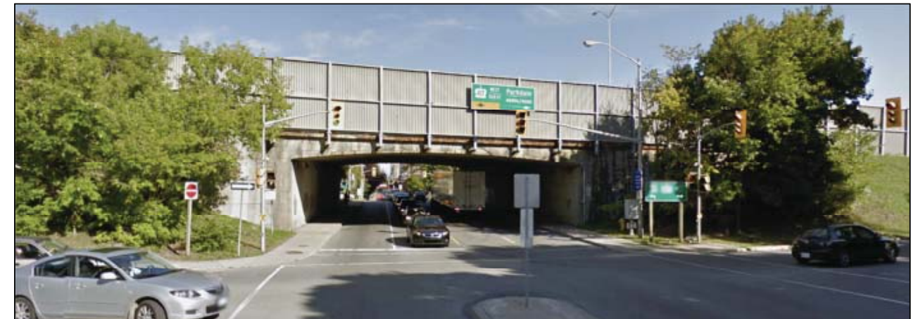
Figure 3. Parkdale Avenue Bridge (looking north)
