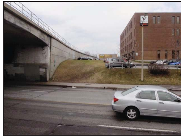
Plate 45: West view of NW quadrant of Highway 417/ Bank Street bridge.
