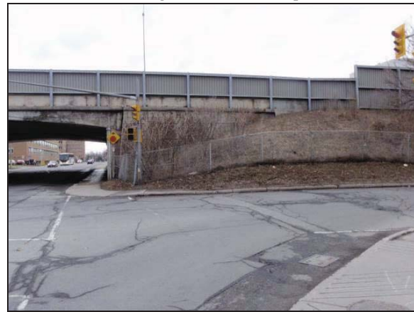
Plate 33: South view of NW quadrant of Highway 417/Booth Street bridge.
