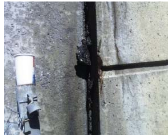
Photo 02: Cork asphalt board in expansion joint
