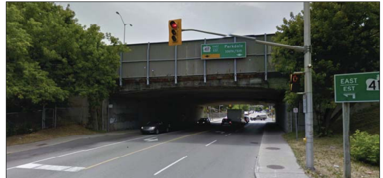
Figure 4. Parkdale Avenue Bridge (looking south)
