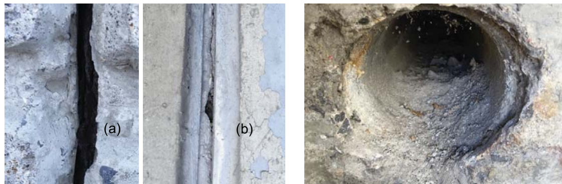
Photo 01: Caulking and mortar in construction joints
