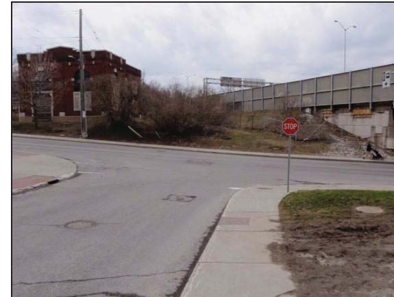
Plate 3: West view hydro sub-station south of the Highway 417/ Holland Avenue bridge.
