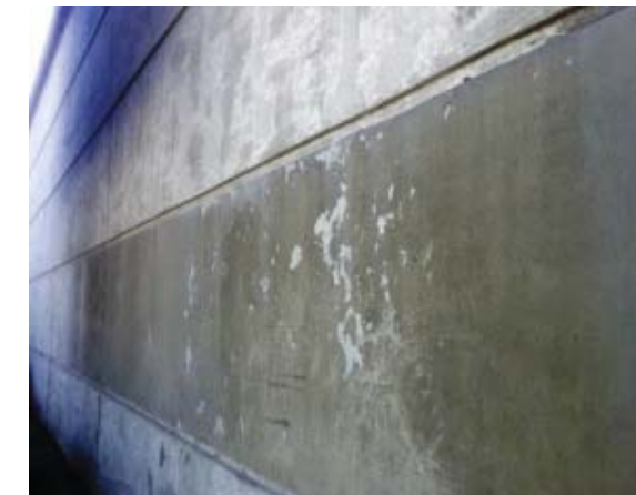
Photo 01: Paint on abutment walls
