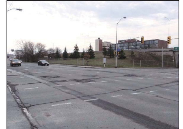
Plate 50: Southeast view of NE quadrant of Highway 417/ O'Connor Street bridge.
