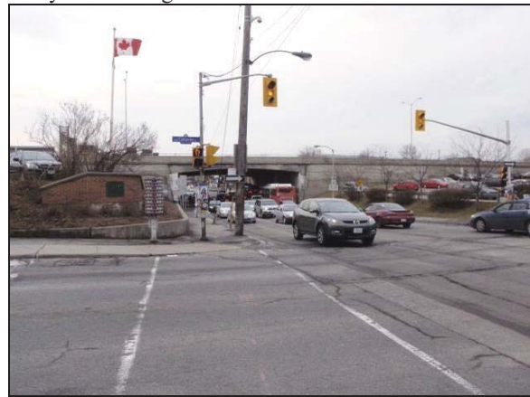
Plate 46: South view of NW and NE quadrant of Highway 417/ Bank Street bridge.
