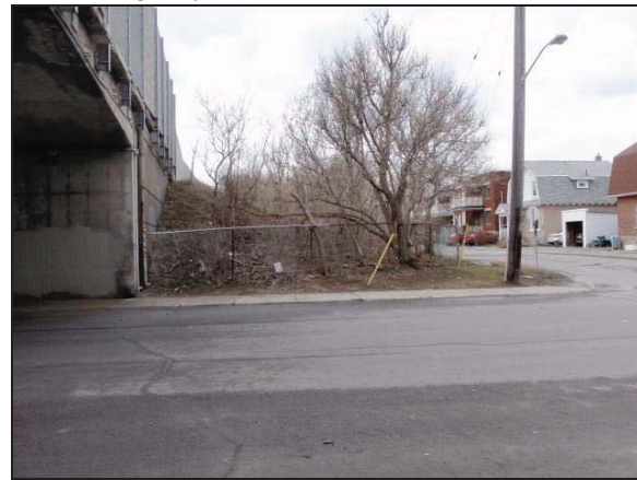
Plate 9: West view of NW quadrant of Highway 417/ Fairmont Avenue bridge.
