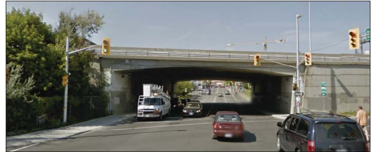
Figure 22. Bank Street Bridge (looking north)
