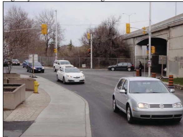
Plate 48: West view of SE quadrant of Highway 417/ Bank Street bridge.
