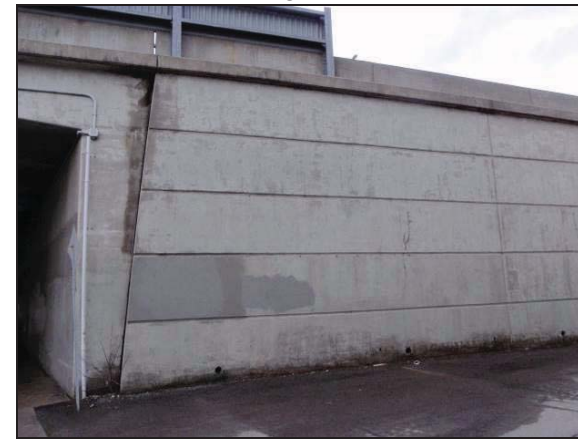
Plate 41: South view of NW quadrant of Highway 417/Percy Street bridge
