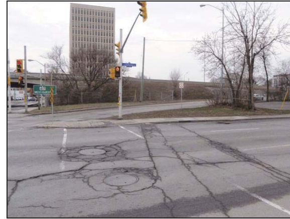
Plate 49: South view of NW quadrant of Highway 417/ O'Connor Street bridge.
