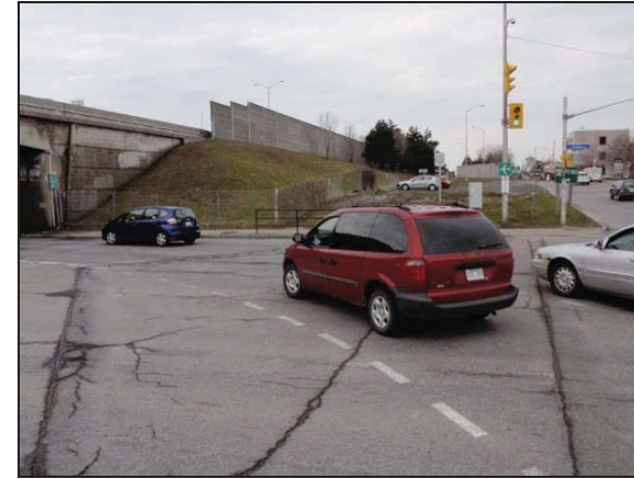
Plate 37: West view of NW quadrant of Highway 417/Bronson Avenue bridge.
