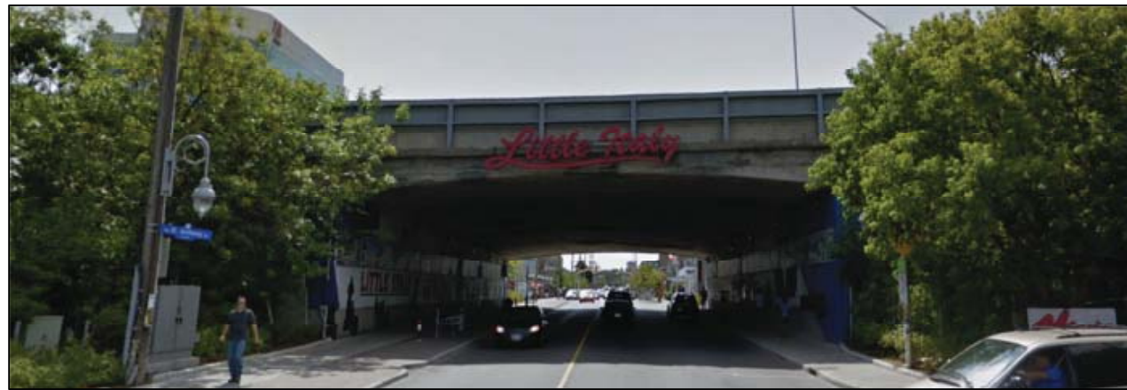
Figure 13. Preston Street Bridge (looking south)
