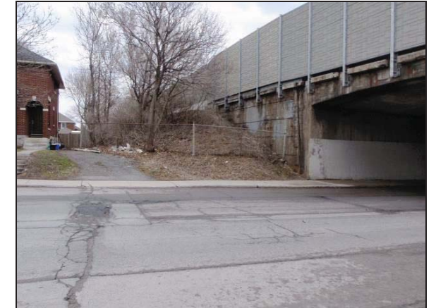
Plate 14: East view of NE quadrant of Highway 417/ Bayswater Avenue bridge.
