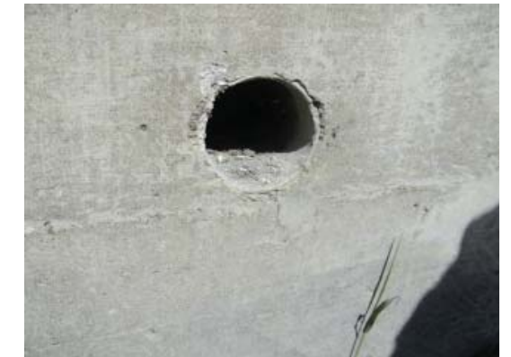
Photo 02: Transite Drainage Duct in Retaining Wall
