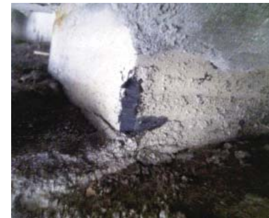
Photo 03: Rubberised Bearing Block
