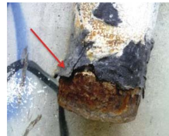
Photo 05: Drain Pipe Coating
