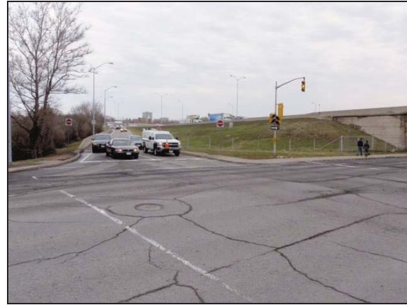
Plate 31: West view of SW quadrant of Highway 417/Rochester Street bridge at EBL exit ramp.
