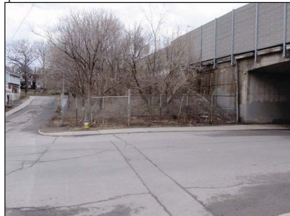
Plate 10: East view of NE quadrant of Highway 417/ Fairmont Avenue bridge.
