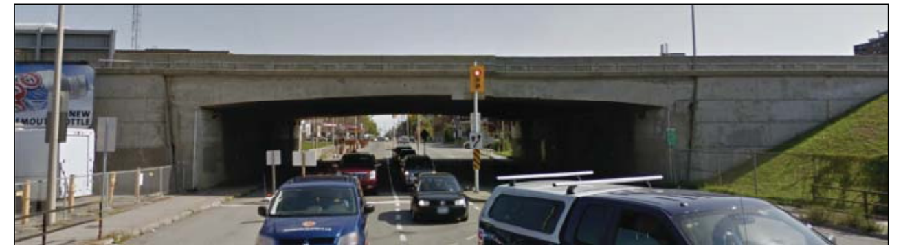
Figure 19. Bronson Avenue Bridge (looking south)
