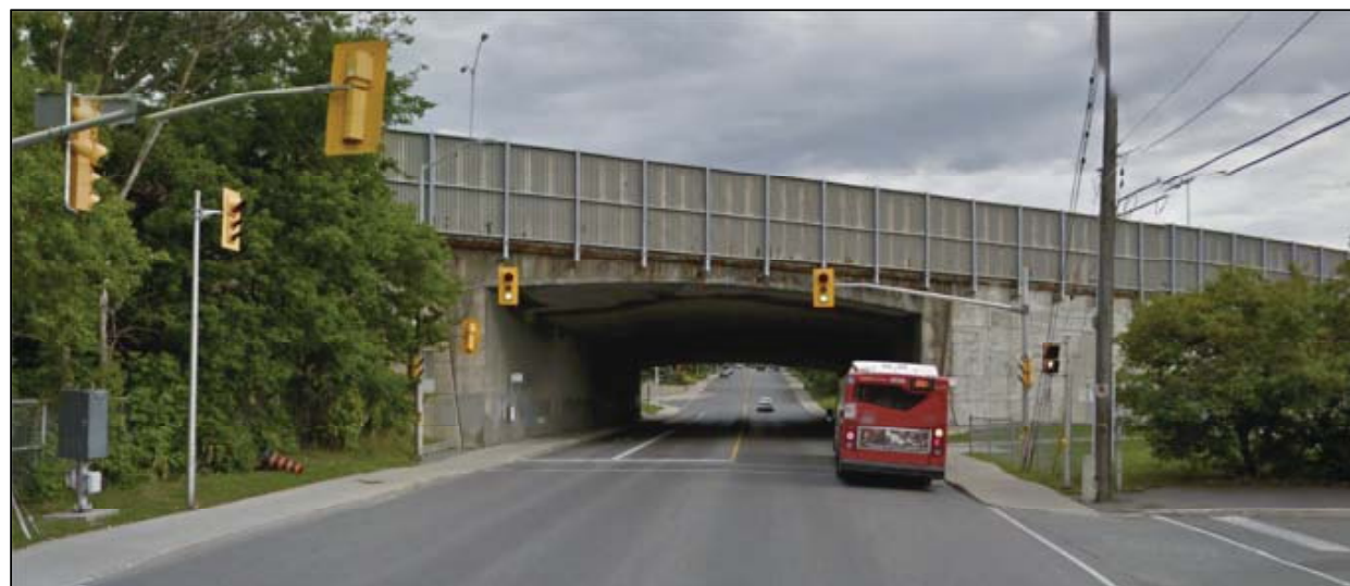
Figure 2. Holland Avenue Bridge (looking south)
