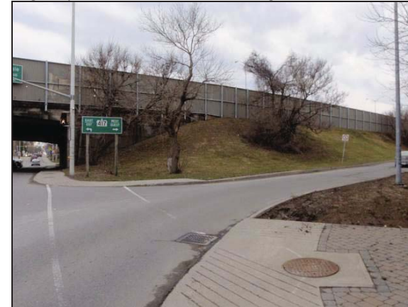
Plate 5: South view of NW corner of Highway 417/ Parkdale Avenue bridge.
